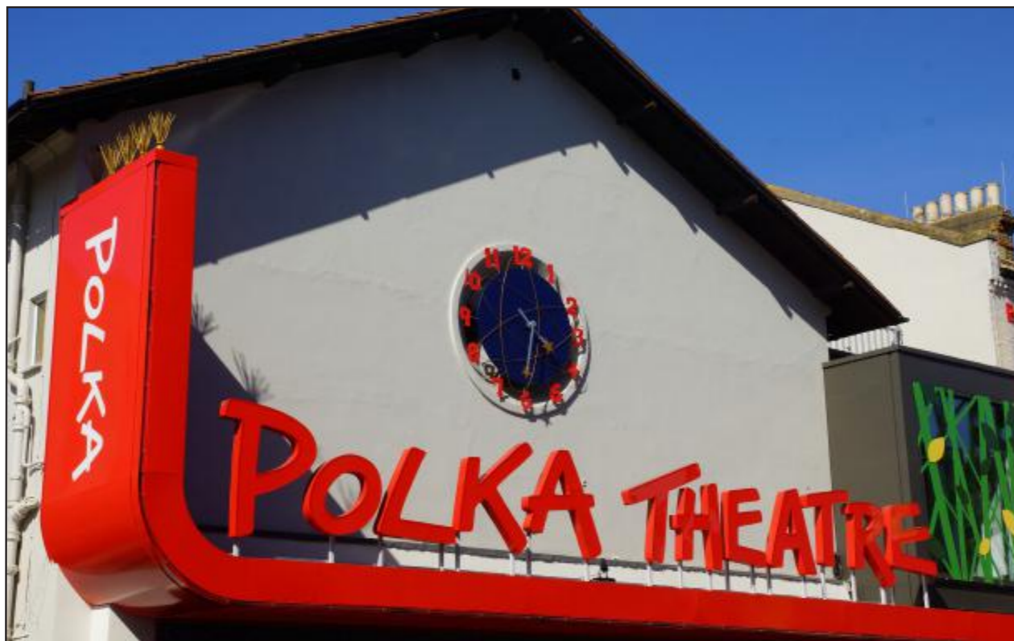
TRANSFORMATION: External picture of Polka Theatre that has taken over a year to build. The now newly renovated building has undergone a major re-development project to celebrate the theatre's 40th anniversary
